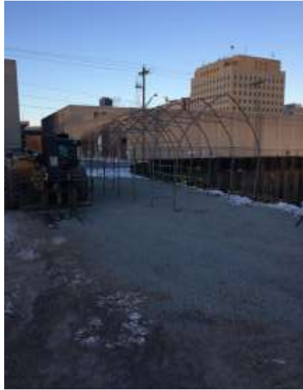
Beginning stages of the temporary shelter to house the grouting machine.
