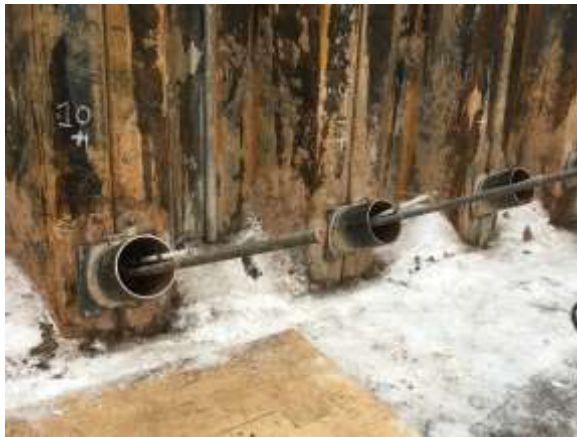
Example of the fully installed earth retention system.
