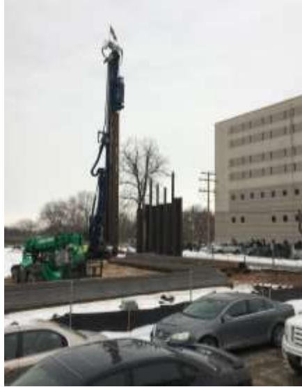
Michels making progress along Eighth Street after the fiber was suspended.
