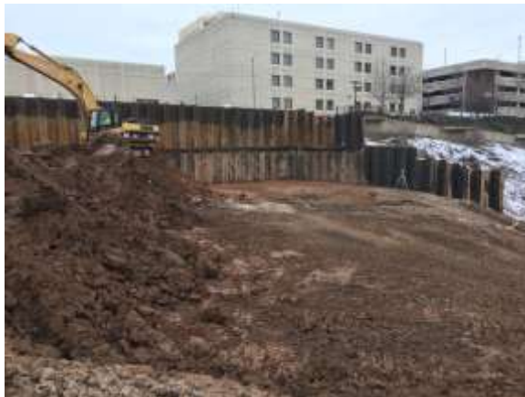
Progress of the Tier 2 excavation along Lawrence Street.
