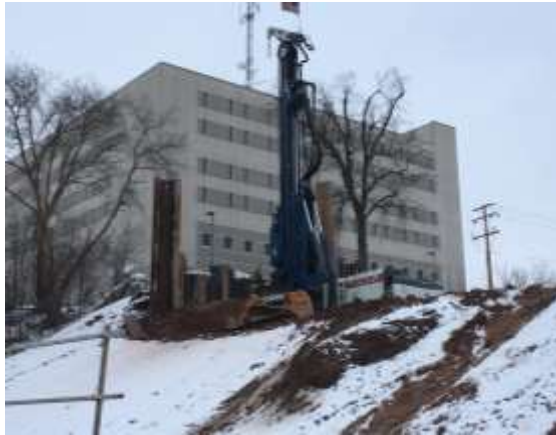
Michels driving the remaining shorter sheet piling into the southeast corner.
