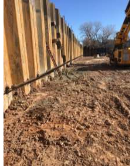
All tiebacks along Lawrence Street have been installed.
