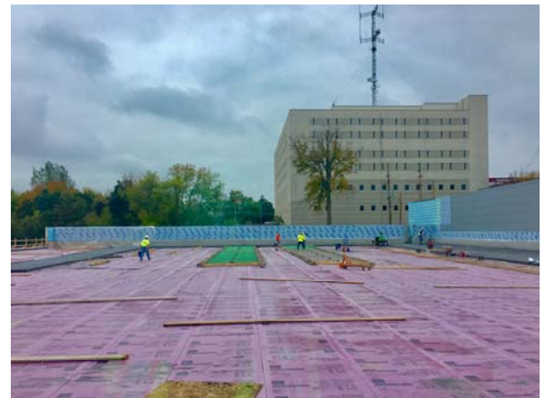
Martell has begun pouring the plaza deck.
