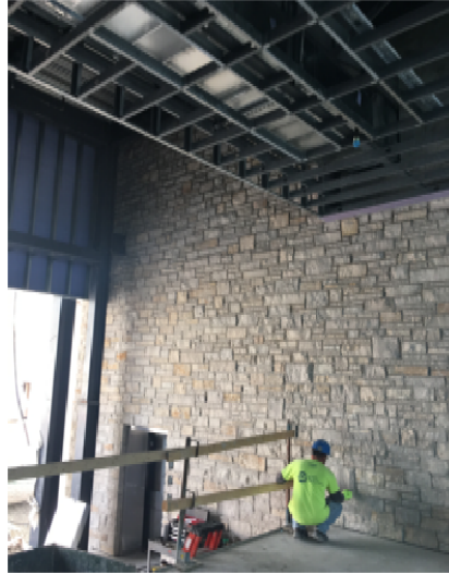
Interior stone at the plaza level nears completion.
