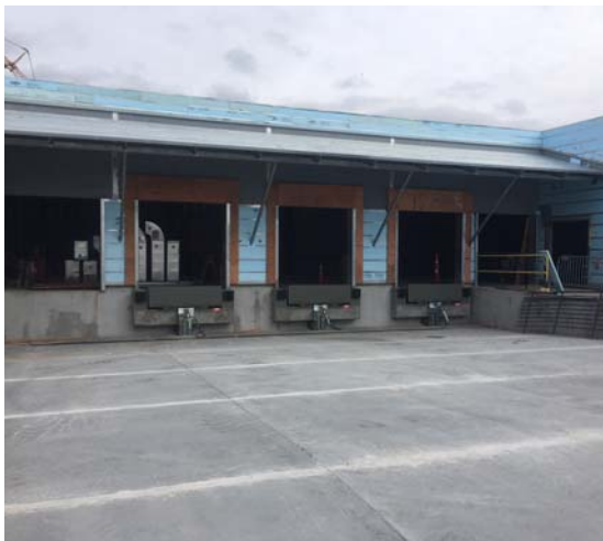
Loading dock equipment is being installed; concrete is complete.
