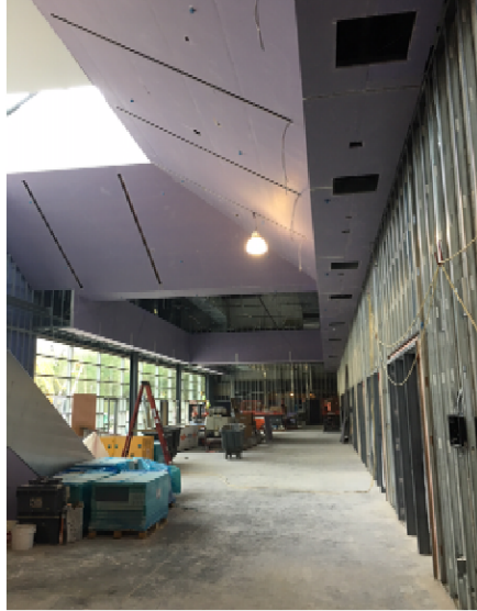
Drywall installation continues on soffits in the pre-function area.
