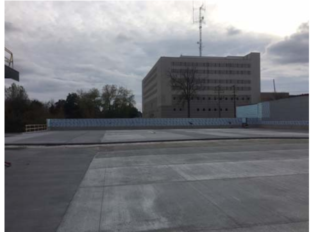
Work continues on the plaza deck concrete.
