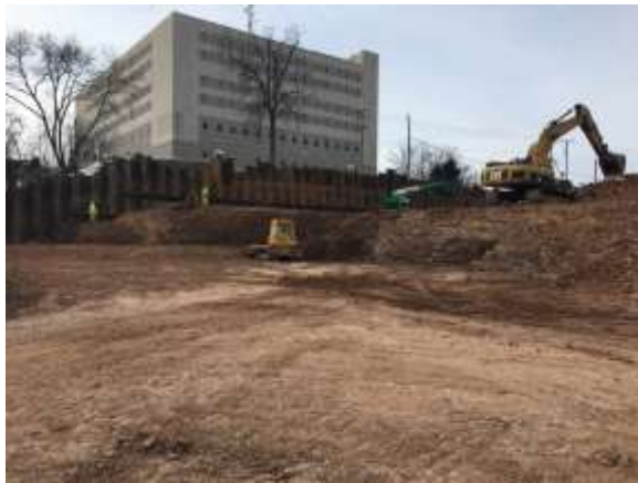
Progress of the Tier 2 excavation along Eighth Street.
