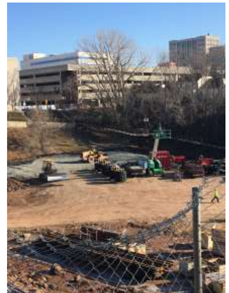
Calnin & Goss installing fabric and stone at the laydown area expansion.
