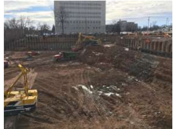
Crews working on the excavation of Tier 2.
