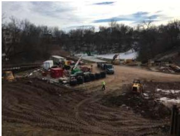
Work being conducted on the additional laydown area.
