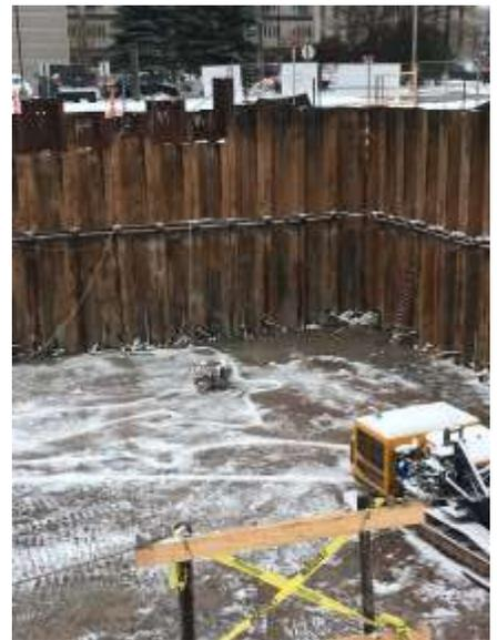
Tiebacks have been installed to the corner of Eighth and Elm Street. Walers will be installed in the coming week.
