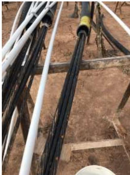
Closer look at the type of tieback anchor being used. Unlike the top tier, the bottom tiers utilize a stranded cable in lieu of a threaded rod.
