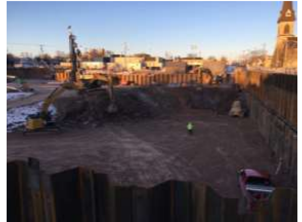
Progress of the tier 2 excavation.
