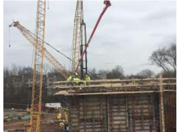
Concrete crew members pouring concrete for the freight elevator shaft walls.
