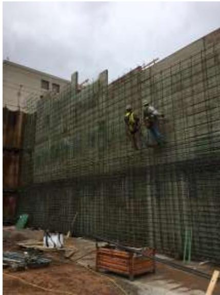
Rebar crew members tying in the final pieces of the rebar cage at the east retaining wall.
