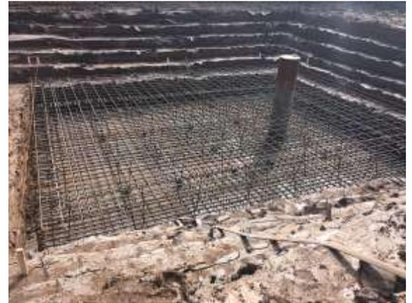
The rebar cage for the freight elevator pit. The pipe in the middle is the hydraulic shaft for the elevator itself.
