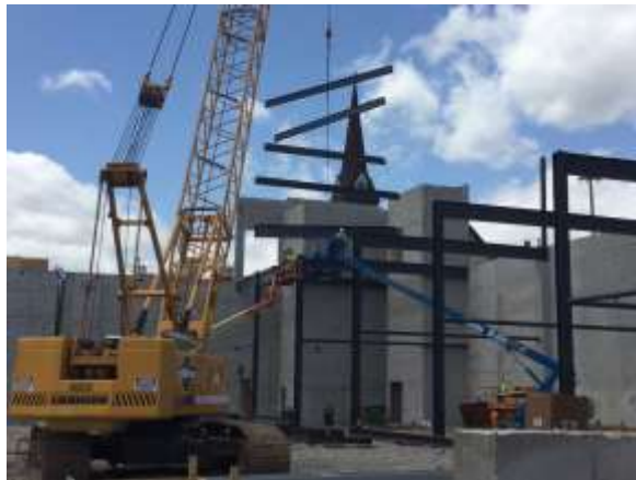
The northwest elevator shaft is complete. Steel erection has begun.
