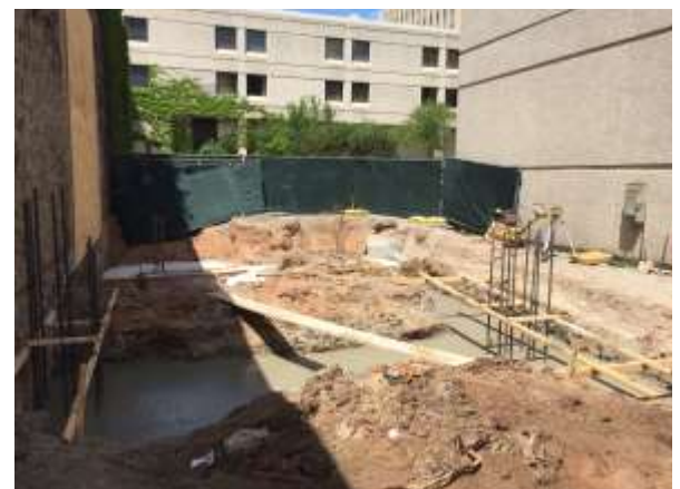
New concrete footings at the Radisson Paper Valley Hotel.
