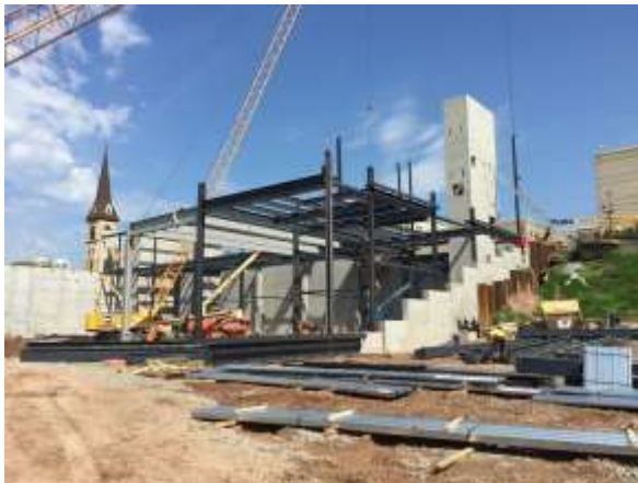
Steel erection continues for the northern portion of FCEC.
