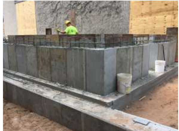
Escalator foundation walls are poured at the Radisson Paper Valley Hotel.
