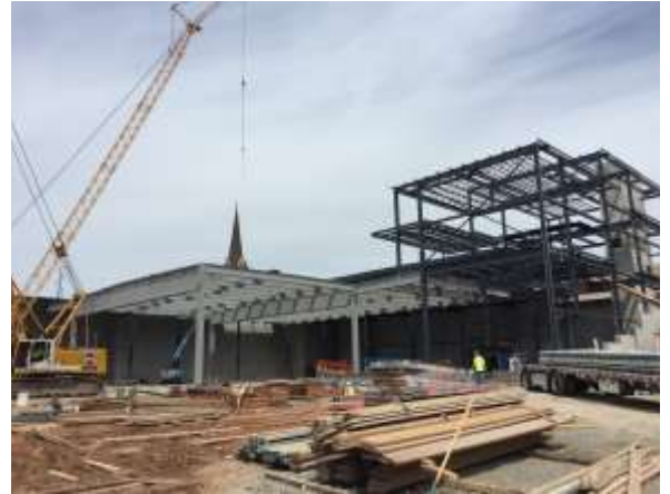
Steel has been set for the exhibition center roof/plaza level.
