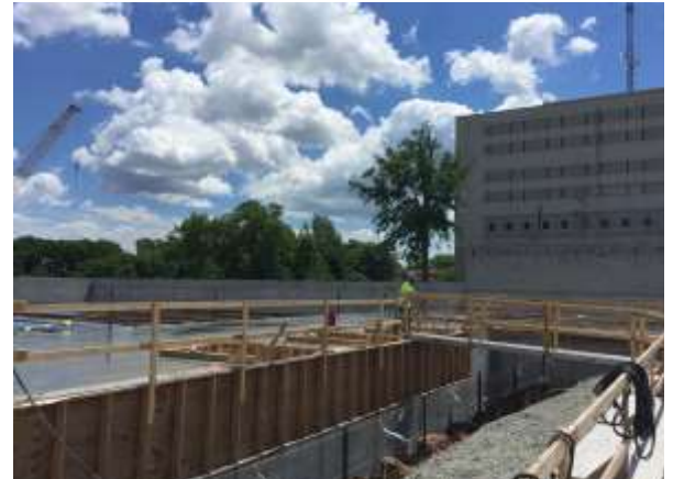
The loading dock deck has been poured.
