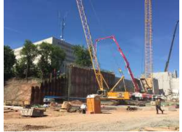
Concrete pour along the south foundation wall.
