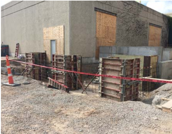
At RPVH: Masons continue work on footings and foundation walls.
