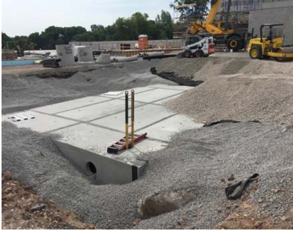
A storm water trap tank was installed.
