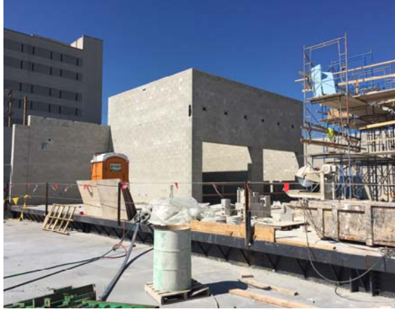
Freight elevator CMU walls are complete.
