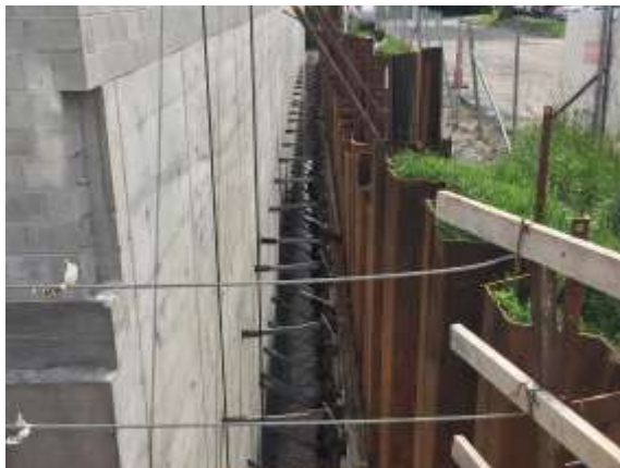
South side of FCEC: tieback installation is almost complete.
